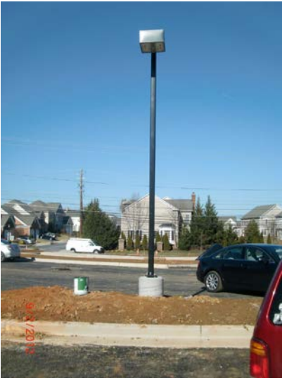
Light pole in the parking lot
