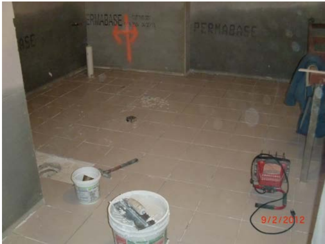
Floor tile in the girl's bathroom
